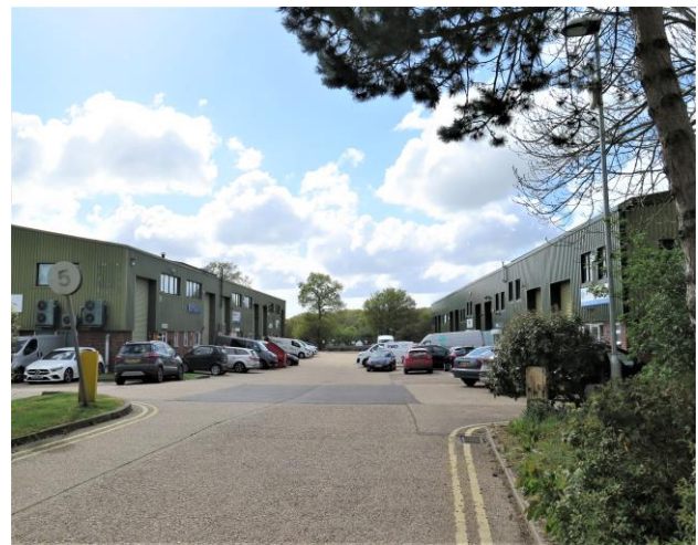
View of Chaucer Business Park
