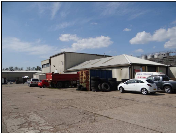
Unit 18 - External View/Parking
