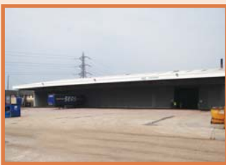
Unit L – Exterior
