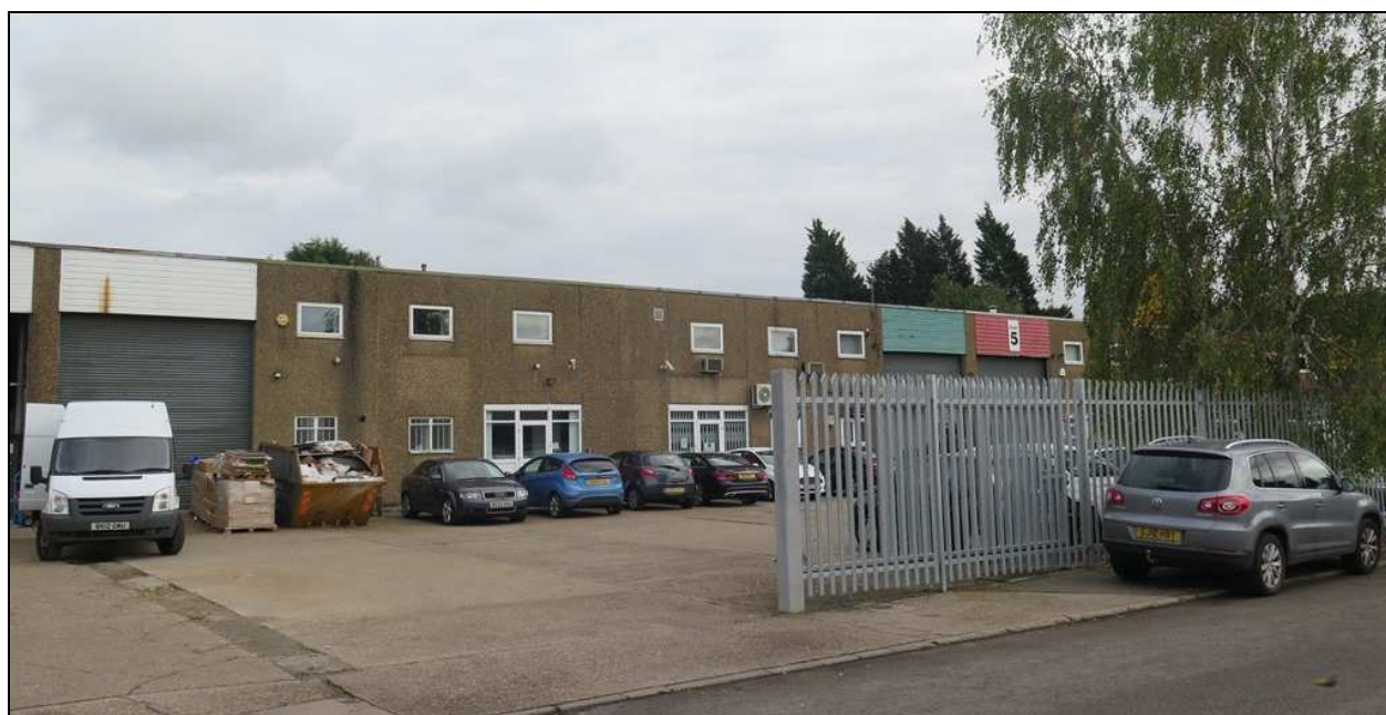
External View of Unit 4
