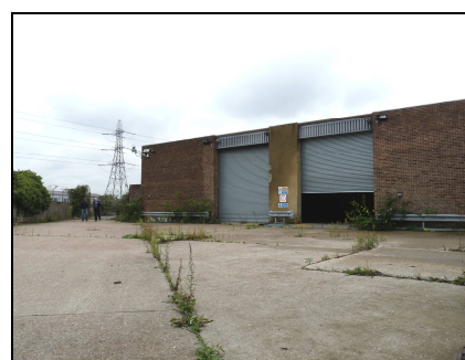
Rear Yard No.2 with Loading Door
