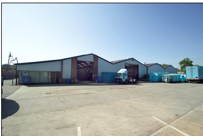
View of Unit 5
