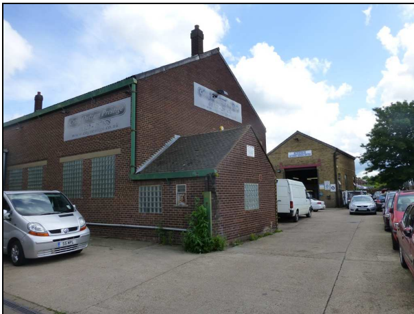
External View of Unit 1
