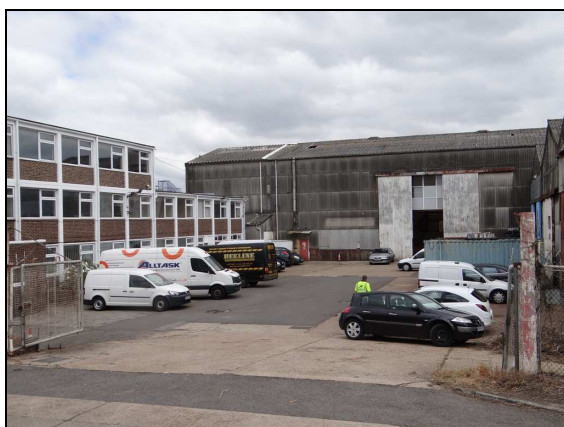
View of Main Yard Area
