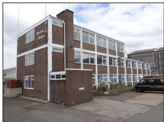
Bowen House Offices
