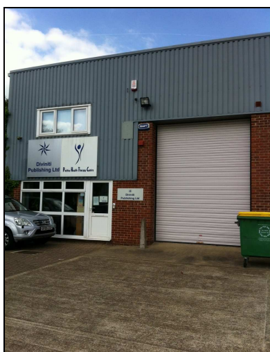
External View of Unit
